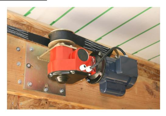
The gears <u>always</u> turn the same speed (2.06 rpm). The problem can be caused by more wraps of the belt on one drum than on the drum on the other side of the house. Even ½ of a wrap can make a difference. It makes a slightly larger diameter drum and therefore a slightly faster belt. This is more noticeable with the longer black belts, because they have more wraps and larger diameters when fully closed.
